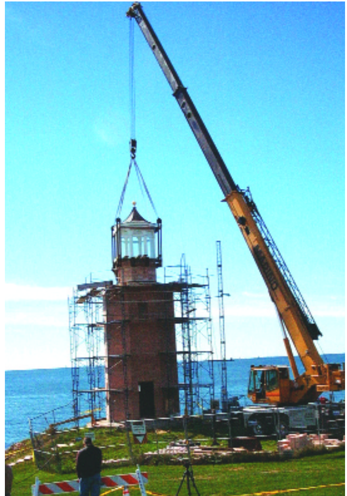
Workers set the restored lantern atop the Avery Point Lighthouse at the UConn campus in Groton, Connecticut, in October, 2005.
