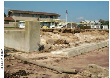
Tropical Storm Irene caused erosion and seawall damage in Fenwick/Old Saybrook.
