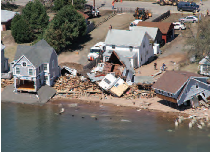
Tropical Storm Irene removed a structure from its pilings at Cosey Beach in East Haven,.
